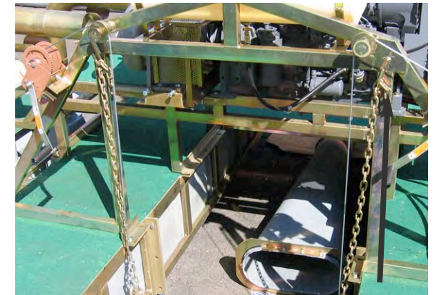
FIG 1I Connect winch and chains to support sluice box ladder.
