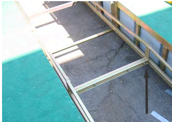
FIG 1H Assemble sluice box ladder to frame and bolt and bolt to rear frame support (Fig 1C).
